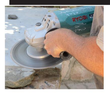
The rear of the rock may be flattened if not flush enough using the side of a diamond tipped blade
