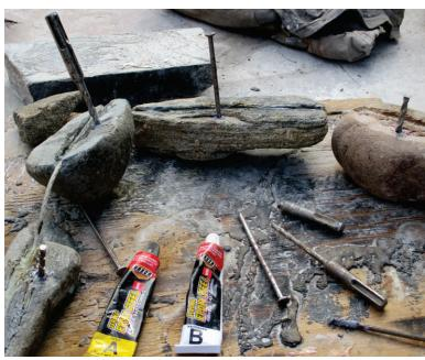
A small hole is drilled from the rear three quarters of the way through and a pin glued in place. The pin may be part of an old drill bit or a nail but preferable something that wont rapidly rust if outside
